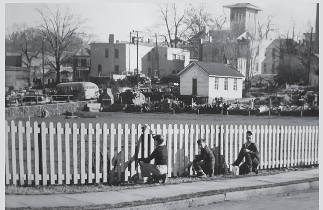
Figure 2. Boy Scouts Painting a Newly Installed Fence at the Memorial Playground in Late 1949-50, with Recently Installed Scout Hut in the Background (Woman's Club Scrapbook, n.d.).
